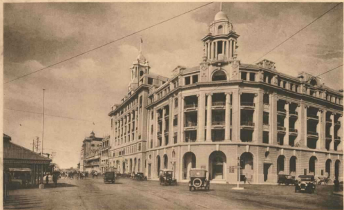
Hongkong-Shanghai Bank and Union Building, Singapore
