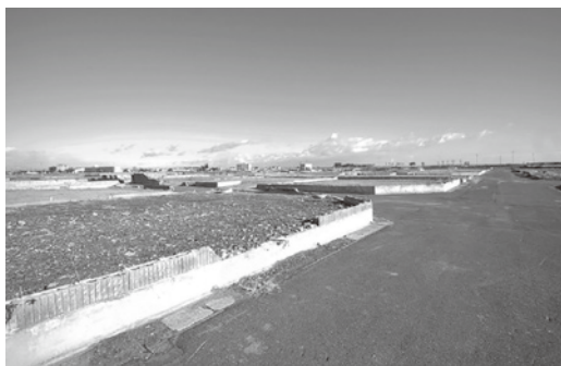
Yuriage area, only foundations of houses were left.
